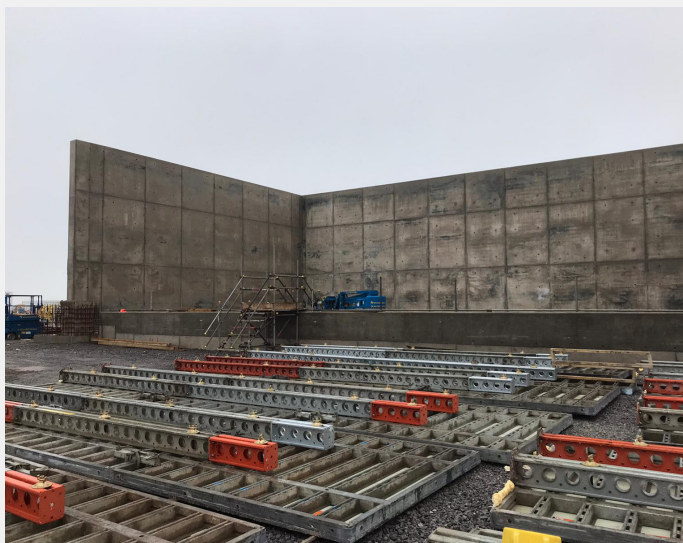
Construction of the new substation at Shurton is progressing well
